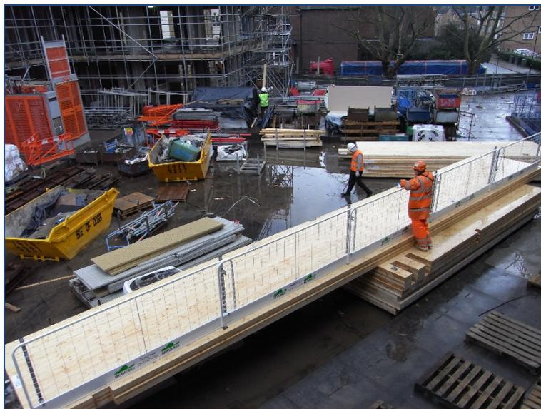
*Figure 1 – CLT Panels as delivered to site.*
