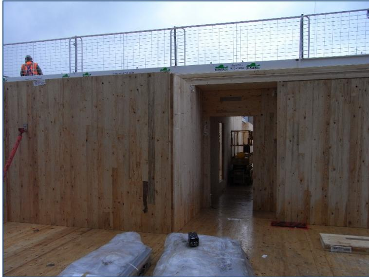
*Figure 2 – CLT Panels in situ.*
